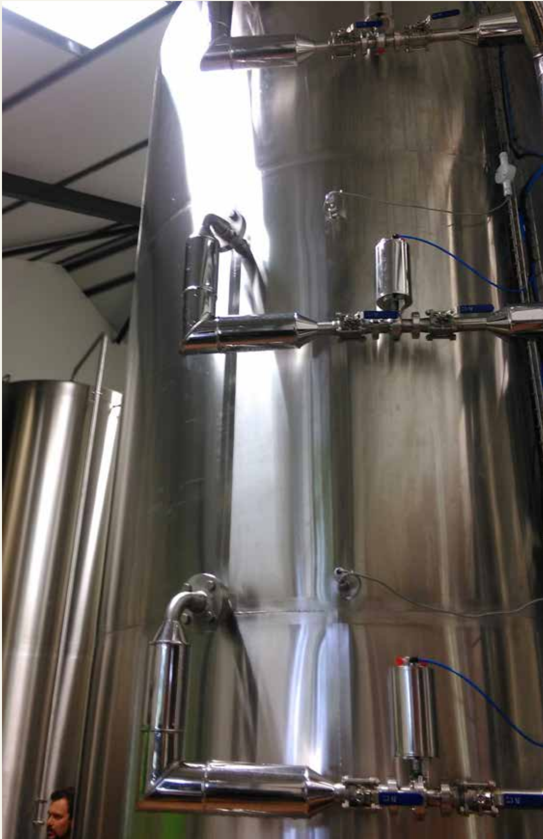
A solar thermal system feeds into a 10 000 litre storage tank at the Cape Brewing Company.
