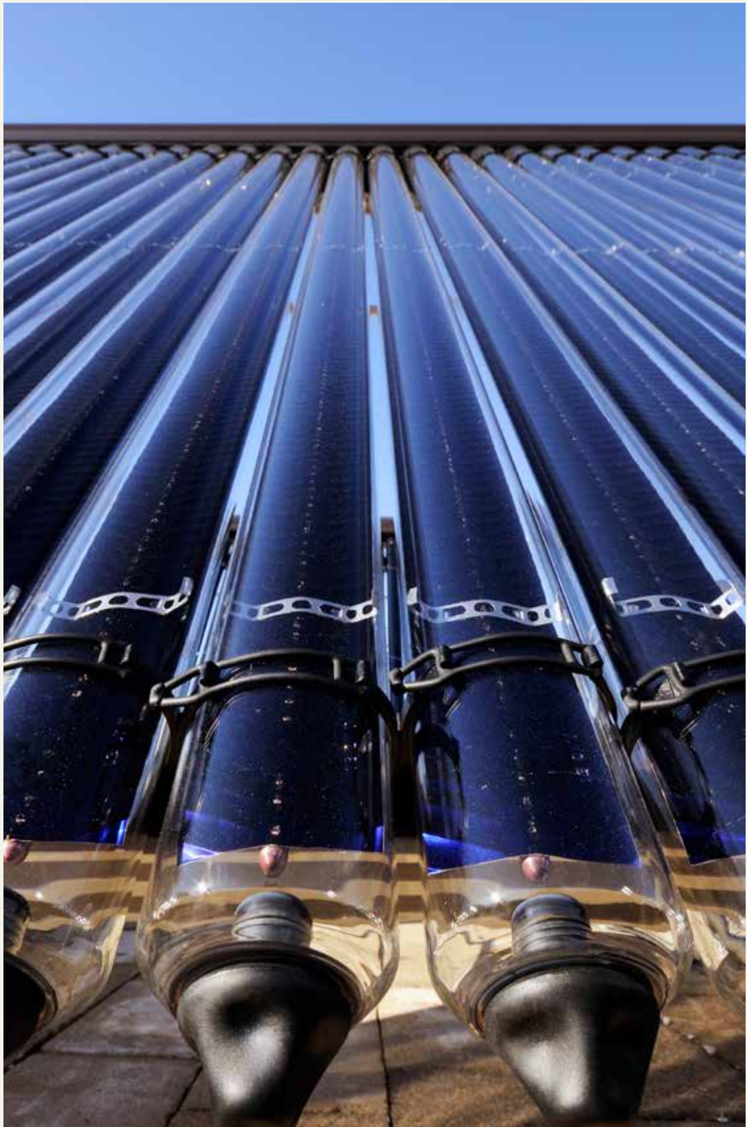
Heat from the sun can be 'captured' in a collector. This photo depicts a non-concentrating evacuated tube collector.
