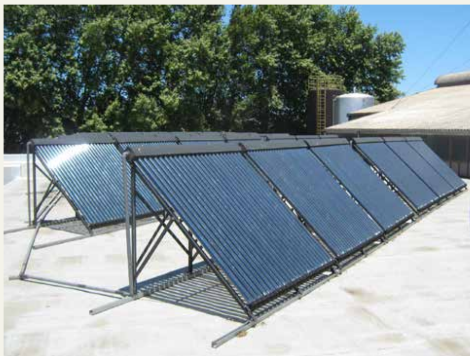
Figure 15: ACA Thread's 156.4m 2 evacuated tube array
