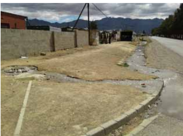
An overflowing manhole in Nduli.
